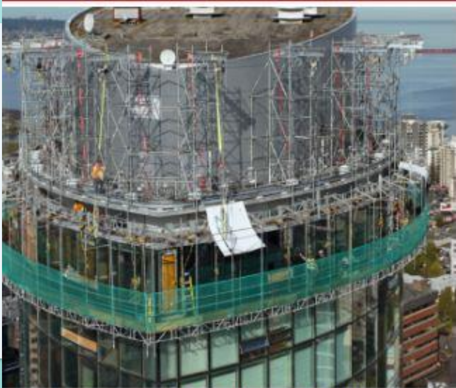
Figure 11: Installed suspended scaffolding and hoist towers
