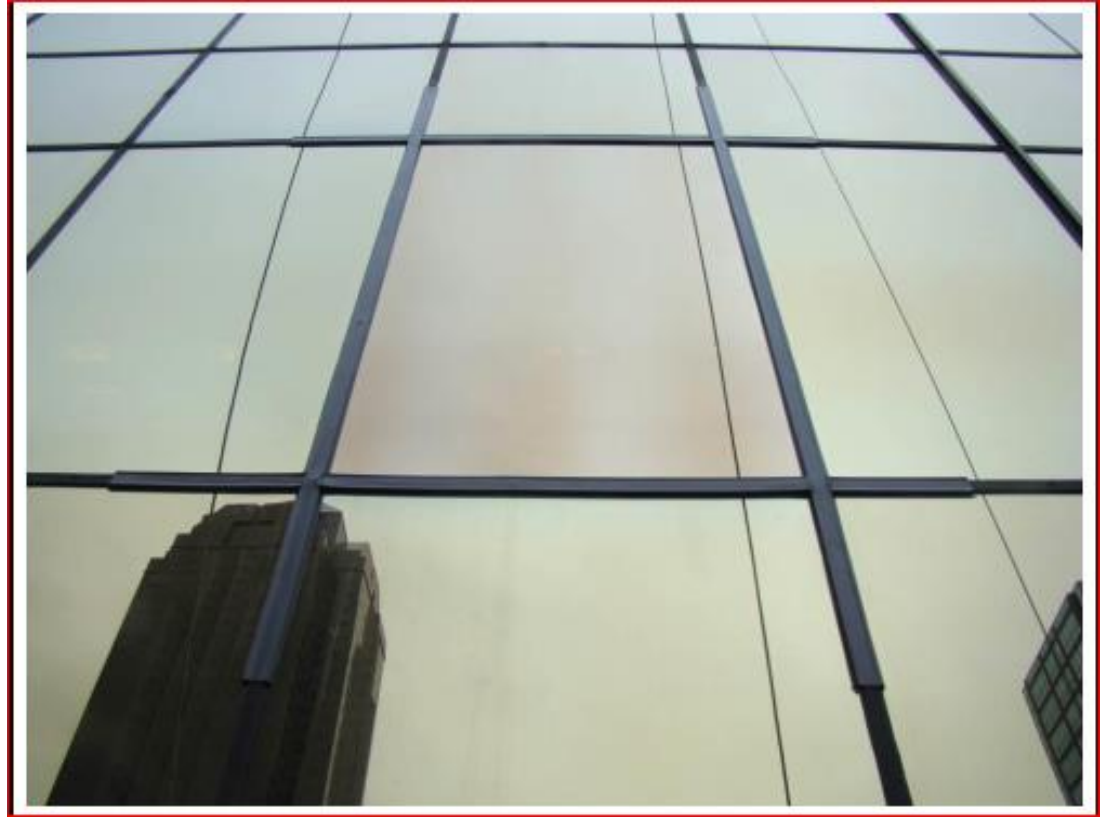
Overlay System Installation...
